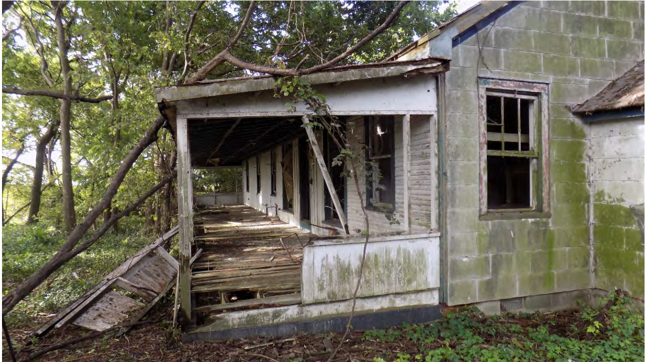
Figure 9. Hunt Club Lodge northeast corner. The eastern exterior, as well as the western and southern exteriors, are covered in white-painted clapboard. Only the northern exterior is covered in asbestos shingles.
