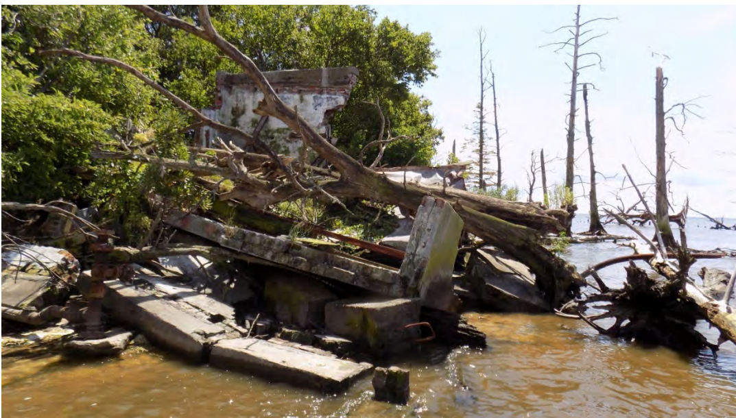
Figure 27. Current state of the generator shed after its collapse due to severe storm events. View looking south.
