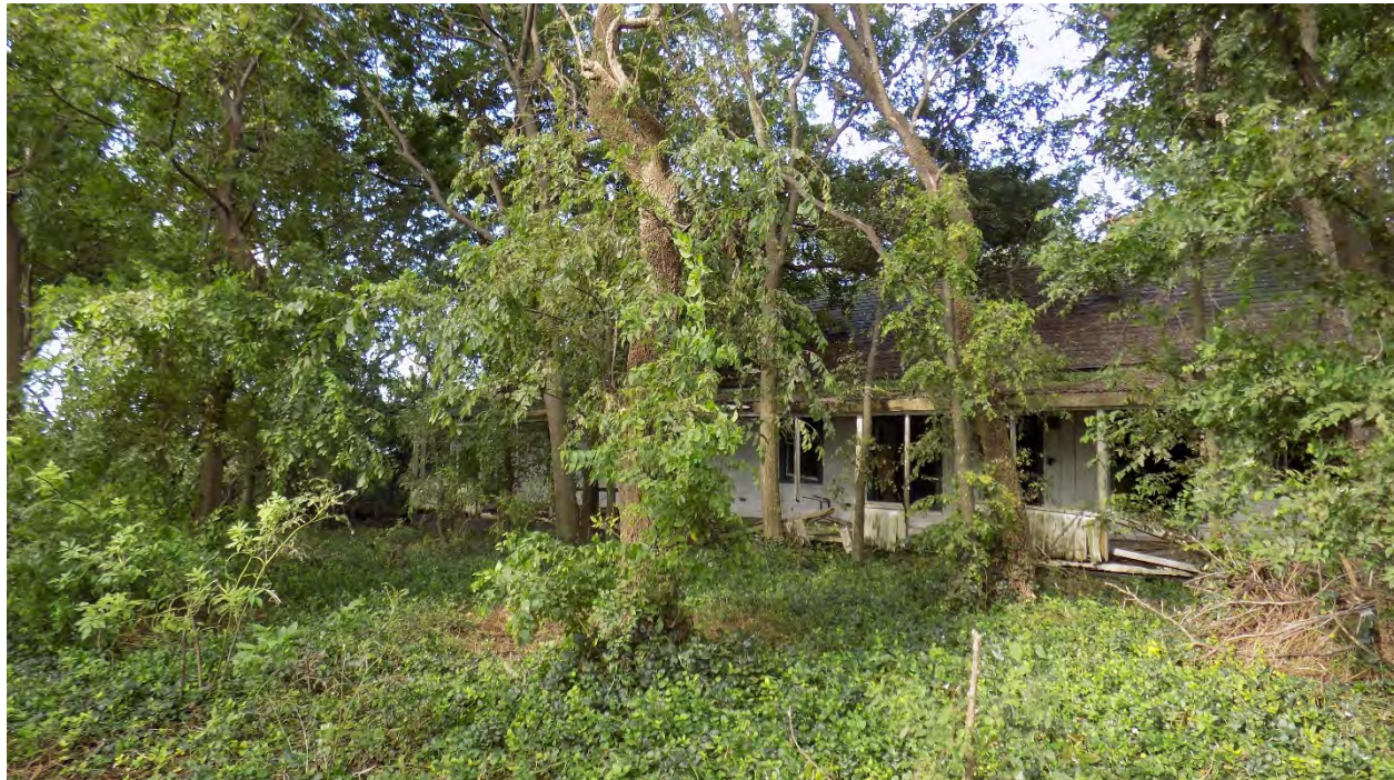
Figure 6. Hunt Club Lodge, eastern elevation. The front deck is in disrepair and foliage has encroached on the structure.
