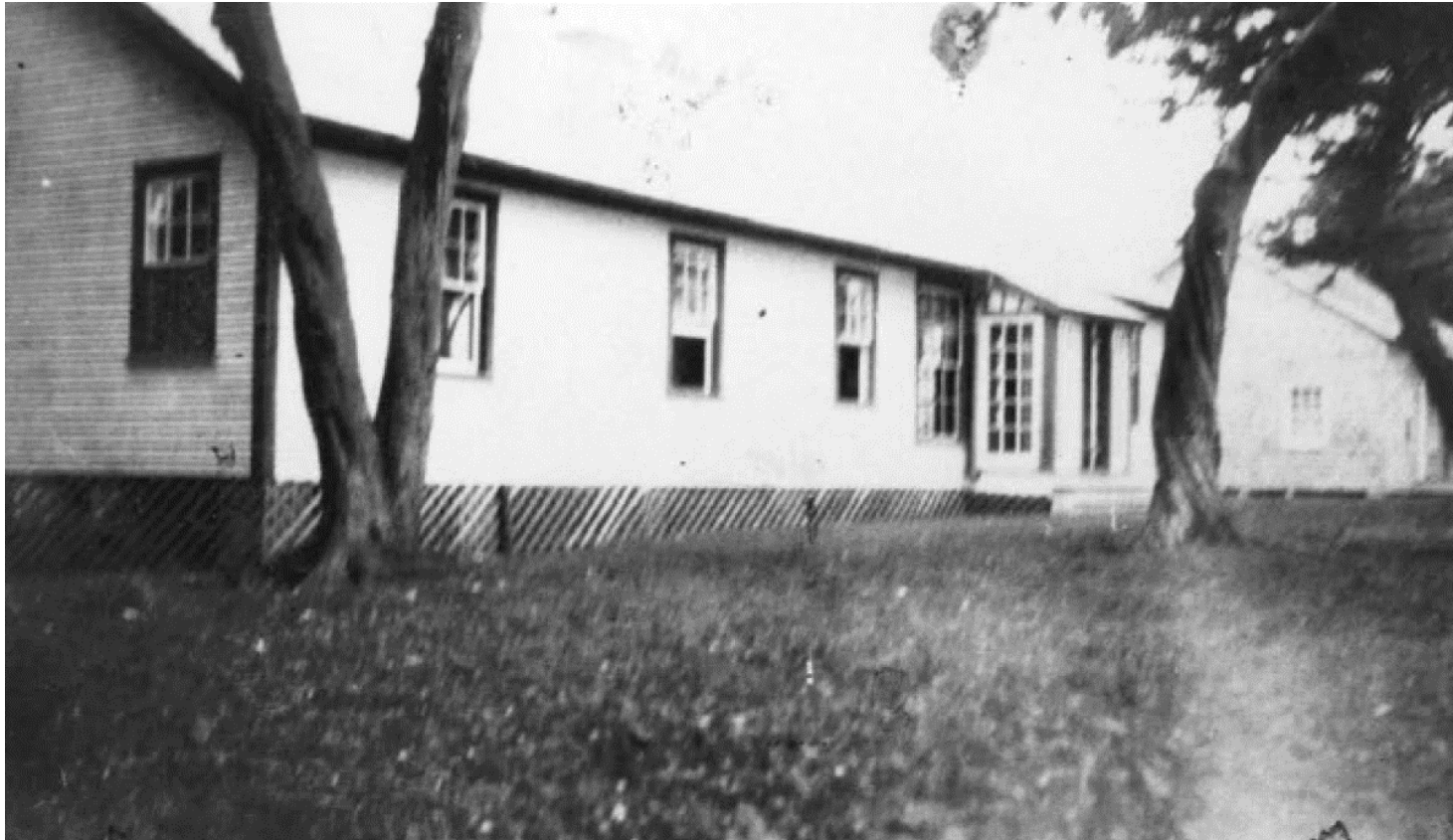
Figure 13. Undated photograph of the Hunt Club Lodge, viewing north-northwest. The picture shows four additional bedrooms to have been constructed extending south of the original footprint. The current existing front deck along this elevation has not yet been constructed (Source: Kanaski [2016]).
