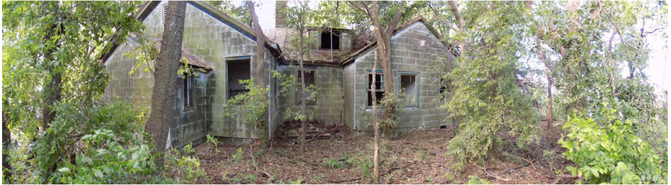
Figure 7. Panorama photograph of the Hunt Club Lodge's northern elevation. The northern exterior wall is the only one to be covered in asbestos shingles. The photograph also depicts the second floor, added bathroom (left), and the remaining northern cistern (middle).
