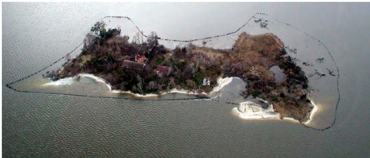
Figure 3. Aerial imagery of Monkey Island from 2005 depicting the location of the Caretaker's Cottage, Hunt Club Lodge, storage shed, boat basin, and retaining wall. Note the significant shoreline erosion due to the failure of the retaining wall (Source: Kanaski [2016]).
