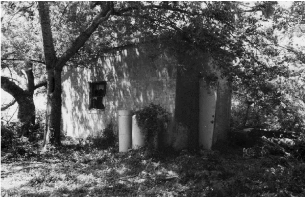
Figure 26. 2001 photograph of the brick and concrete generator shed, southwest corner (Source: Kanaski [2016]).
