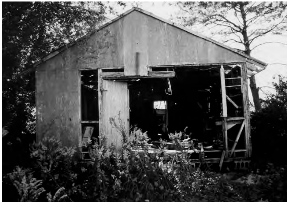
Figure 29. Plywood equipment shed, east elevation, 2001.
